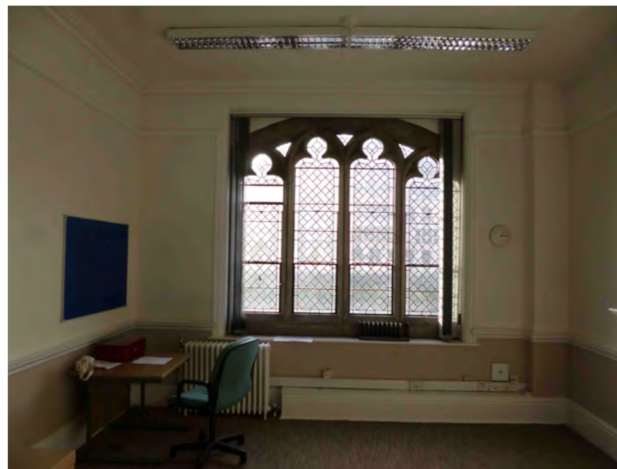
Typical windows in Council Chambers to receive secondary glazing
