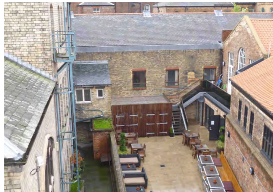
The south east wall of the North Annex with three windows overlooking Jamie's yard
