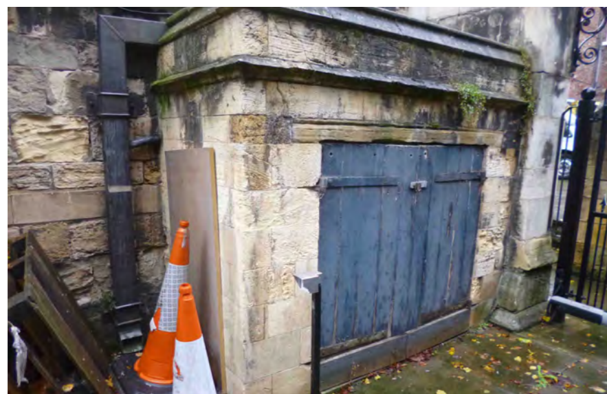
Stone work at the back of the store indicates an earlier opening through the wall at this location. Building materials could be stored in the flood-prone rooms in the basement of the Council Chambers.
