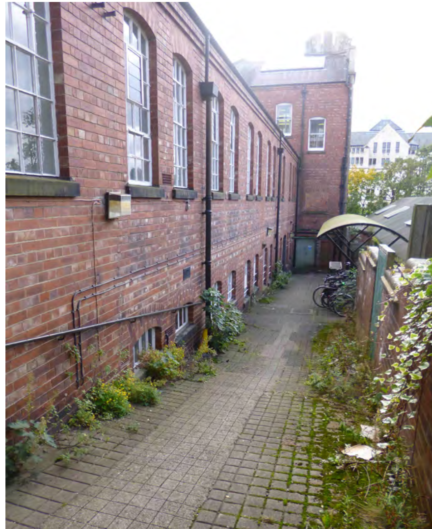
The existing brick rear extension of the North Annex
